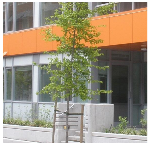
EXTERNAL TREATMENT OF PARKADE WALLS
