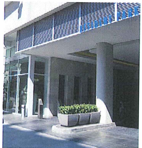
Architectural Integrated Parkade Entry
