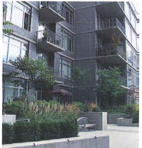
Universally Accesible Main Entrance
