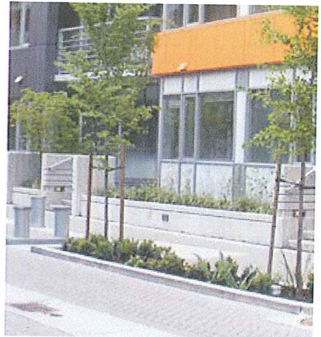
External Treatment of Parkade Walls
