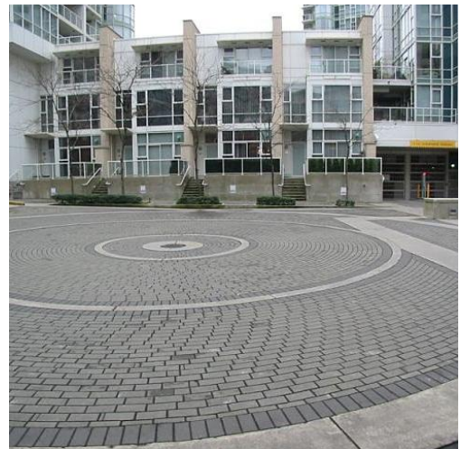
CONSOLIDATED LOADING AND PARKING
