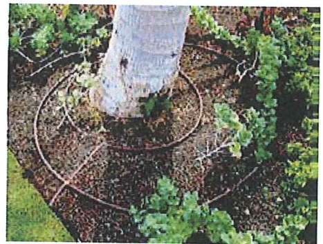
Street Tree Drip Irrigation
