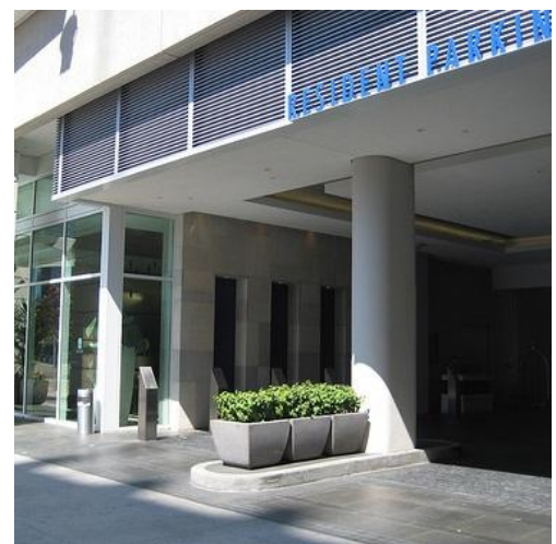
ARCHITECTURAL INTEGRATED PARKADE ENTRY
