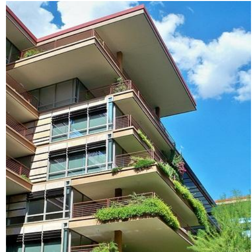
BALCONY AND OVERHANG RESPOND TO CLIMATE
